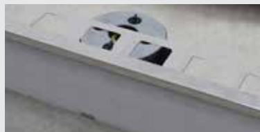
E5. Wedge the cut tile between the BSJ profile and the SUPACLPB clip.
