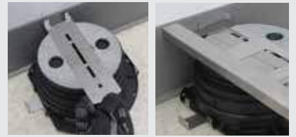
D3. Place the SUPACLPP spacer clip and the BSJ profile on the head of the pedestal.
