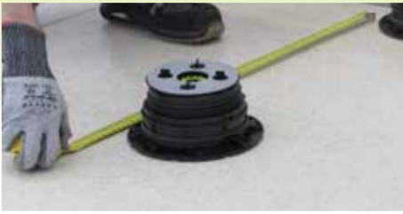
12. Place the center of the pedestals at the same distance as the dimension of the tile. The spacing should not exceed 60 cm on center.
