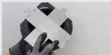
F1. Place two SUPACLPB clips perpendicular to each other under the pedestal base.
