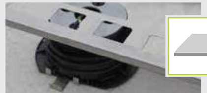
E3. Place the BSJ profile between the tabs on the head of the pedestal.
