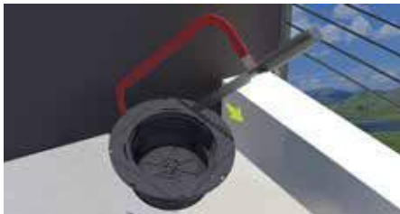
1. Cut one side of the pedestal.
