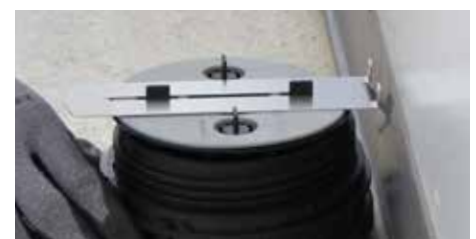
9. Insert a SUPACLPP spacer clip between the two tabs perpendicular to the wall.
