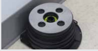
D1. Place the pedestal with one cut side against the wall and the other facing outwards.
