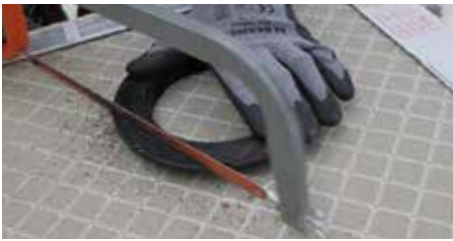
17. Turn the base upside down and remove one of the sides along the marked line.
