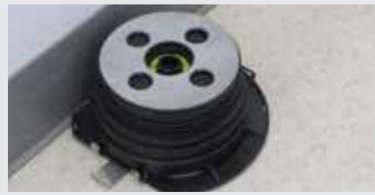
D2. Place the pedestal with one cut side against the wall and the other facing outwards.
