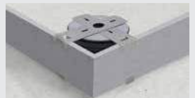
F5. Wedge the cut tile between the SUPACLPT clip and the SUPACLPB clip.
