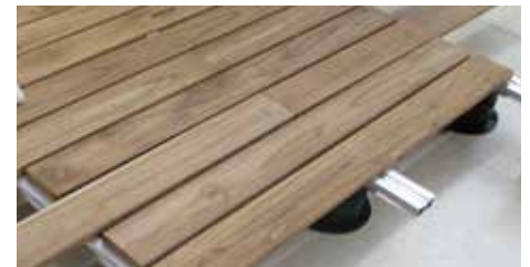
22. Position all the wood boards, inserting the grooves in the SUPCLIP clips.
