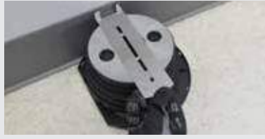
D2. Place the SUPACLPP spacer clip on the head of the pedestal.
