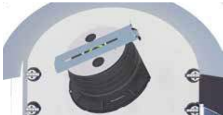
7. Place the SUPACLPP perpendicular to the wall.
