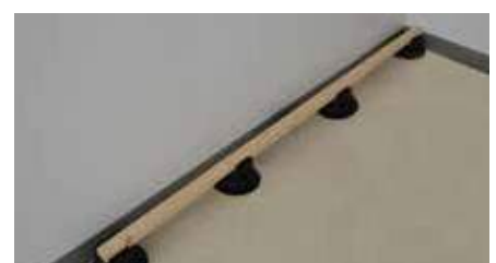
7. Check to make sure that the wood joists are firmly attached to each pedestal.
