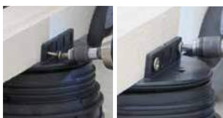
6. Screw the wood joist to the pedestal through the specific slots (use a screwdriver).
