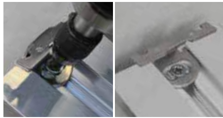
18. Attach the clip to the joist with a screwdriver.
