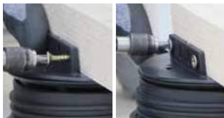
20. Screw the wood joist to the pedestal through the specific slots (use a screwdriver).
