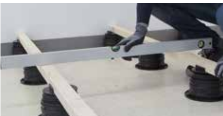
22. Check to make sure that the installation is leveled.
