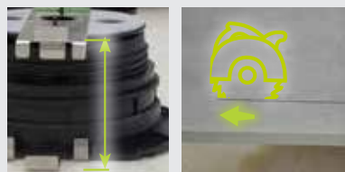
E4. Cut the tile. The dimension of the tile is equal to the distance between the SUPACLPT clip and the SUPACLPB clip.
