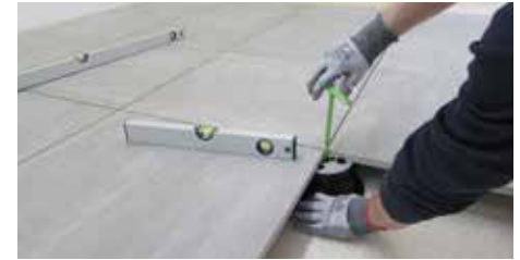
17. If it is not leveled, adjust the height with the SUPAK tool.
