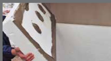
insulation board adhesive
